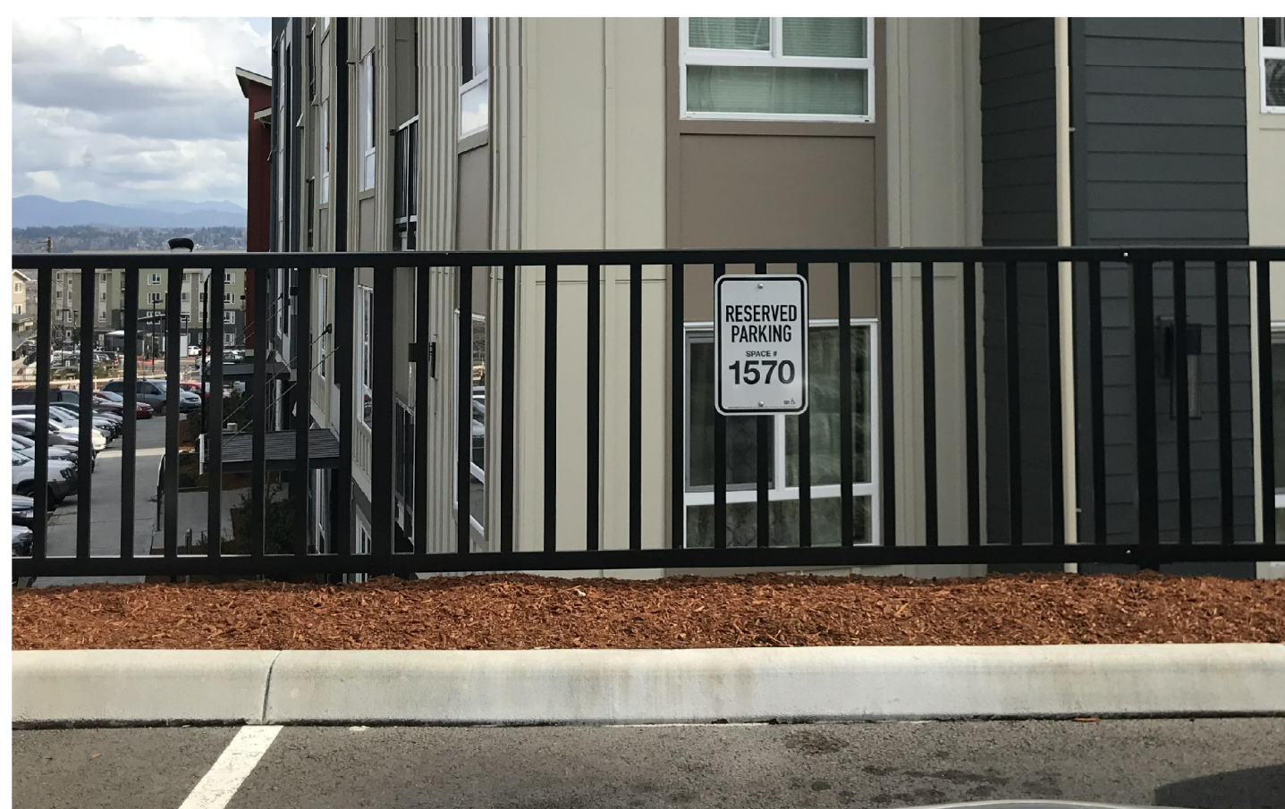
METAL GUARDRAIL FENCE
